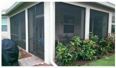
The term under-truss refers to the areas that are underneath a structural part of the home or apartment. A typical condo-style lanai or patio will have an under-truss screen enclosure, where there is a concrete block surrounding the entire area that will be screened.
