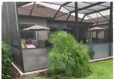
It can also be called a privacy screen. This screen is water-resistant and has a special opaque vinyl coating (almost like plastic) which gives a little more privacy. It's also great at keeping out dirt and debris when placed at the bottom of the enclosure.
