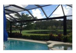
A clearview or picture window is a great way to get rid of all the clutter of normal pool cages that keeps you from truly enjoying the outdoors. It is a high strength aluminum structure that is designed to handle more weight than the average enclosure, which removes almost all vertical beams to wherever clearview is used.
