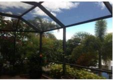
A solar screen can be used to screen entryways. If it used for an under roof application or under-truss screen enclosures, it offers some privacy. This mesh also blocks more than 75% of harmful ultraviolet rays.
